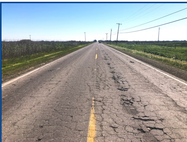
Henry Miller Avenue Rehabilitation Project before
