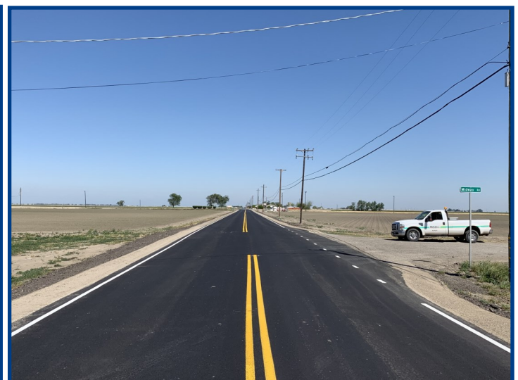
Henry Miller Avenue Rehabilitation Project after
